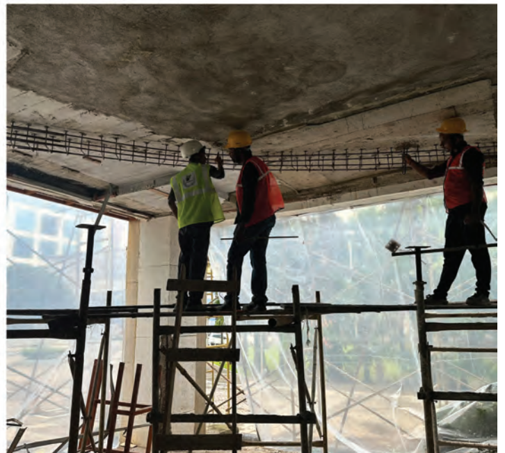
Curve Beam Made To Support The Existing Slab By Using TMT Steel Anchoring(Hilti) And Micro Concrete
