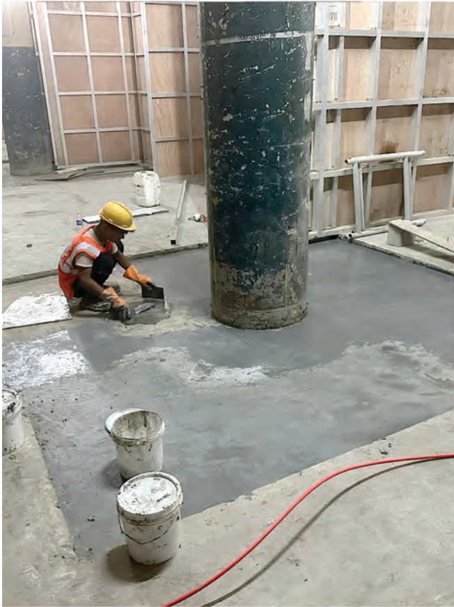
Base Plate Installation To Achieve The Required Strength In Existing Structure.
