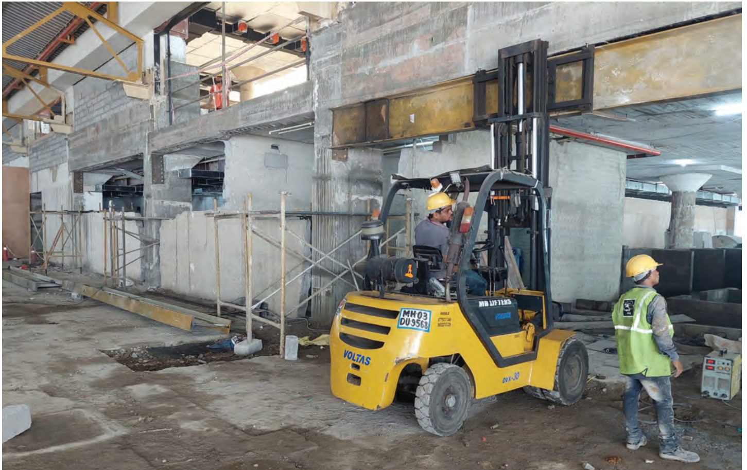
Demolished Tie Beam Strengthening By MS Beam Using Hilti Anchor Fastener & Duct Slab With Ms Fabrication Work
