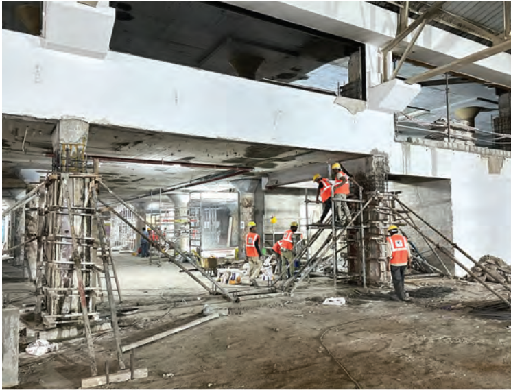
Column Jacketing LV Grout And Micro Concrete.
