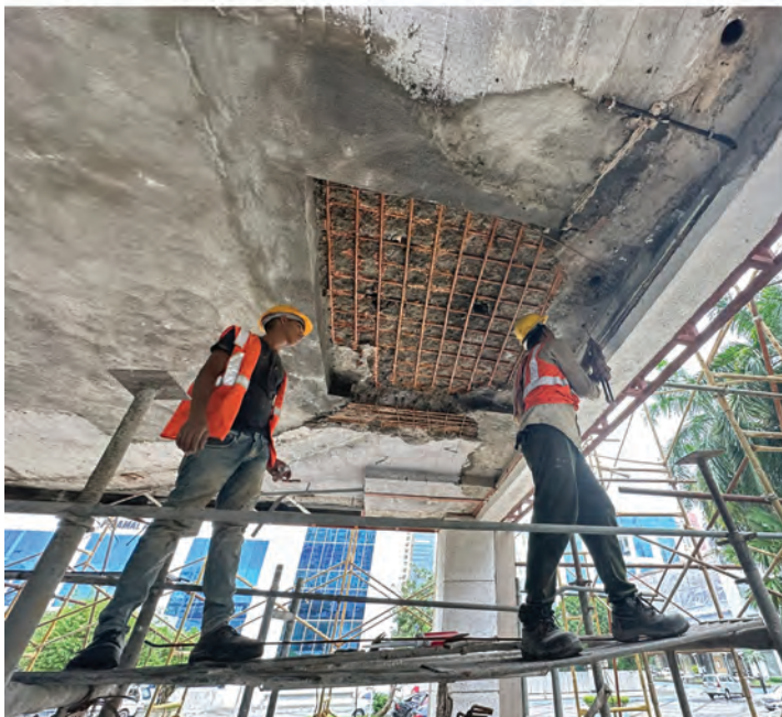
Curve Beam Made To Support The Existing Slab By Using TMT Steel Anchoring(Hilti) And Micro Concrete
