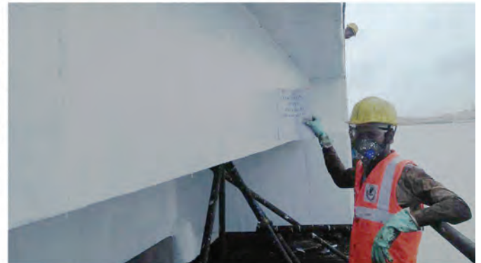
Structure Repair Work For Submerged Area Including Carbon Fiber Wrapping With Anti-carbonation Coating.
