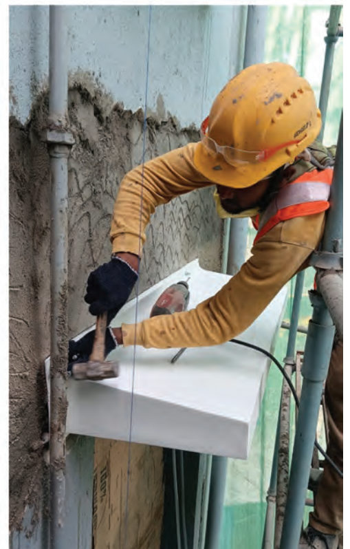
Building Repair Work Done With FRP Chajja
