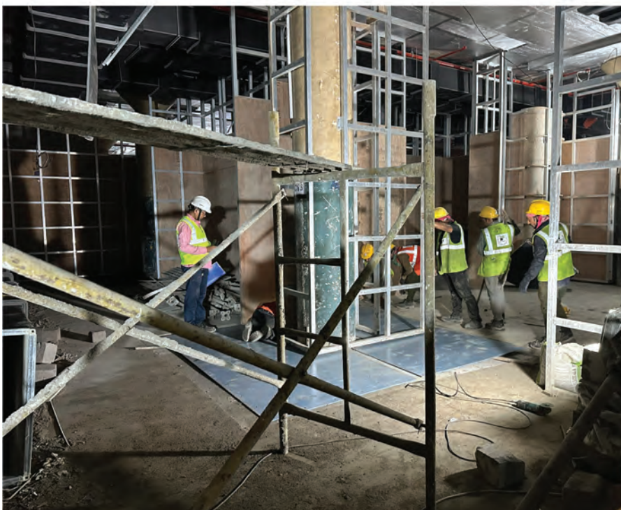
Base Plate Installation To Achieve The Required Strength In Existing Structure.
