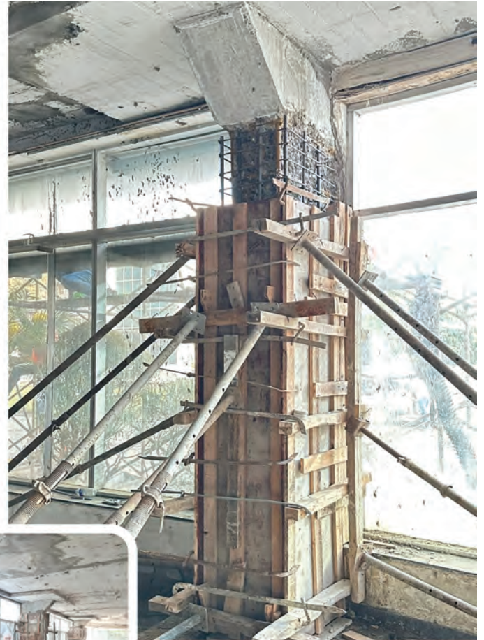
Column Jacketing LV Grout And Micro Concrete.
