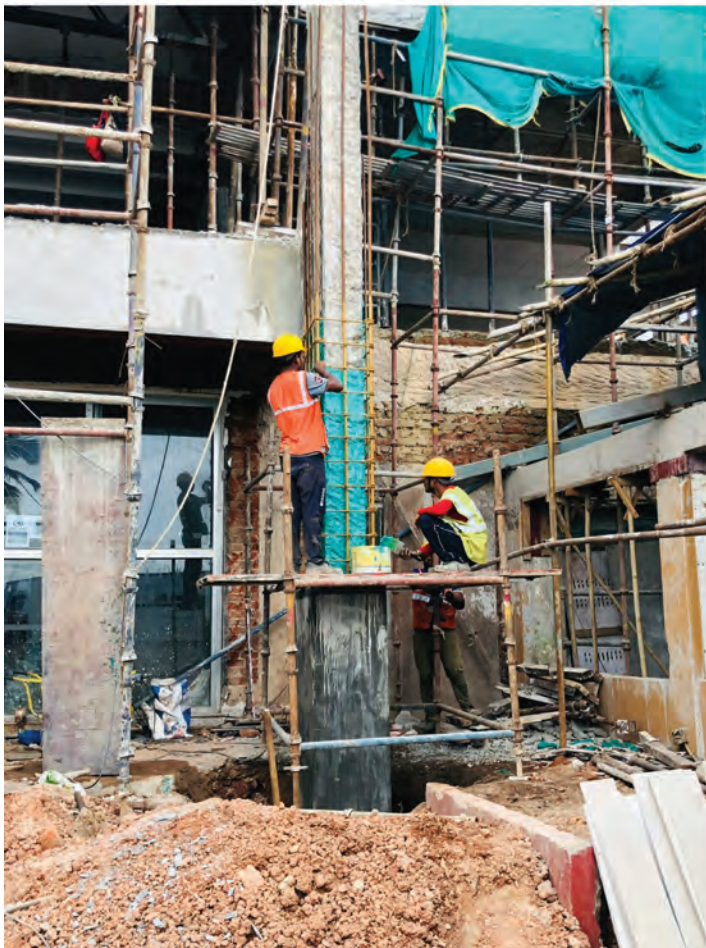
Facade Repair And Column Jacketing Work
