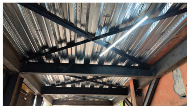
Demolished Tie Beam Strengthening By MS Beam Using Hilti Anchor Fastener & Duct Slab With Ms Fabrication Work
