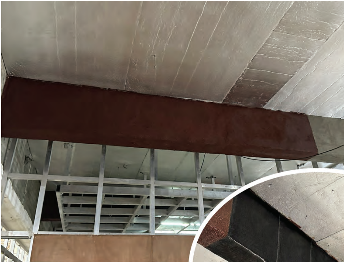
Beam & Column Strengthening Work By Carbon Fiber Wrapping.
