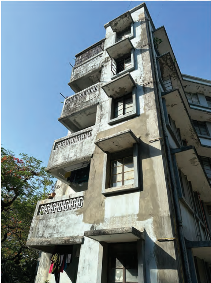
Building Repair Work Done With FRP Chajja
