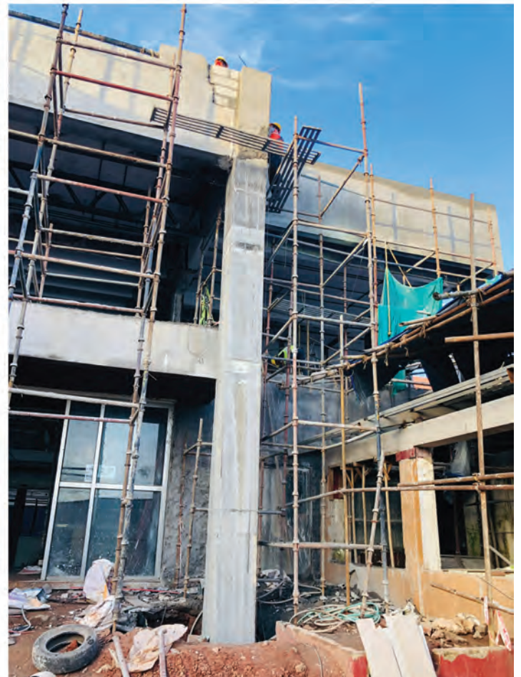
Facade Repair And Column Jacketing Work
