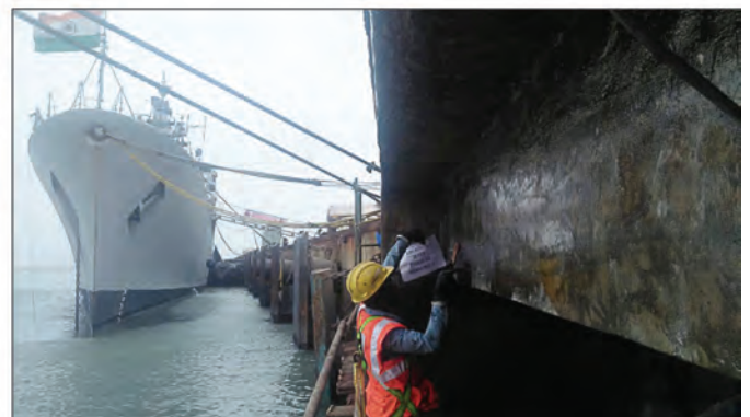
Structure Repair Work For Submerged Area Including Carbon Fiber Wrapping With Anti-carbonation Coating.
