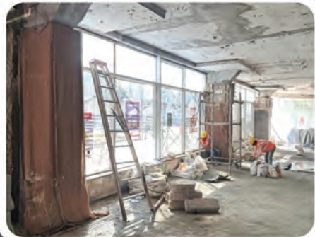
Column Jacketing LV Grout And Micro Concrete.
