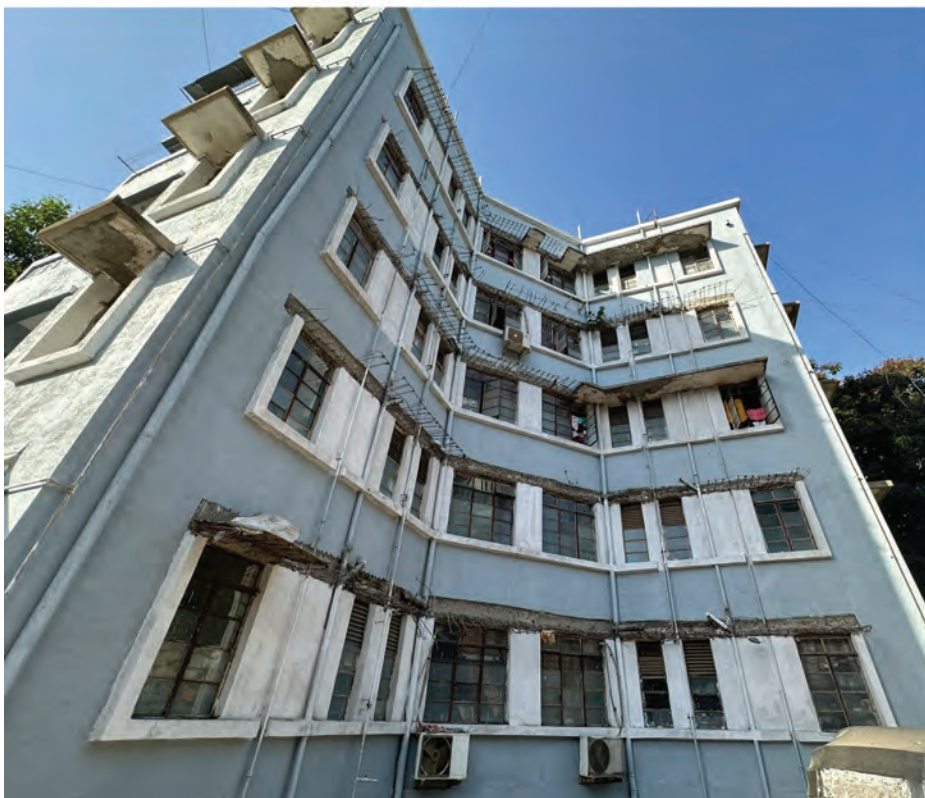
Building Repair Work Done With FRP Chajja
