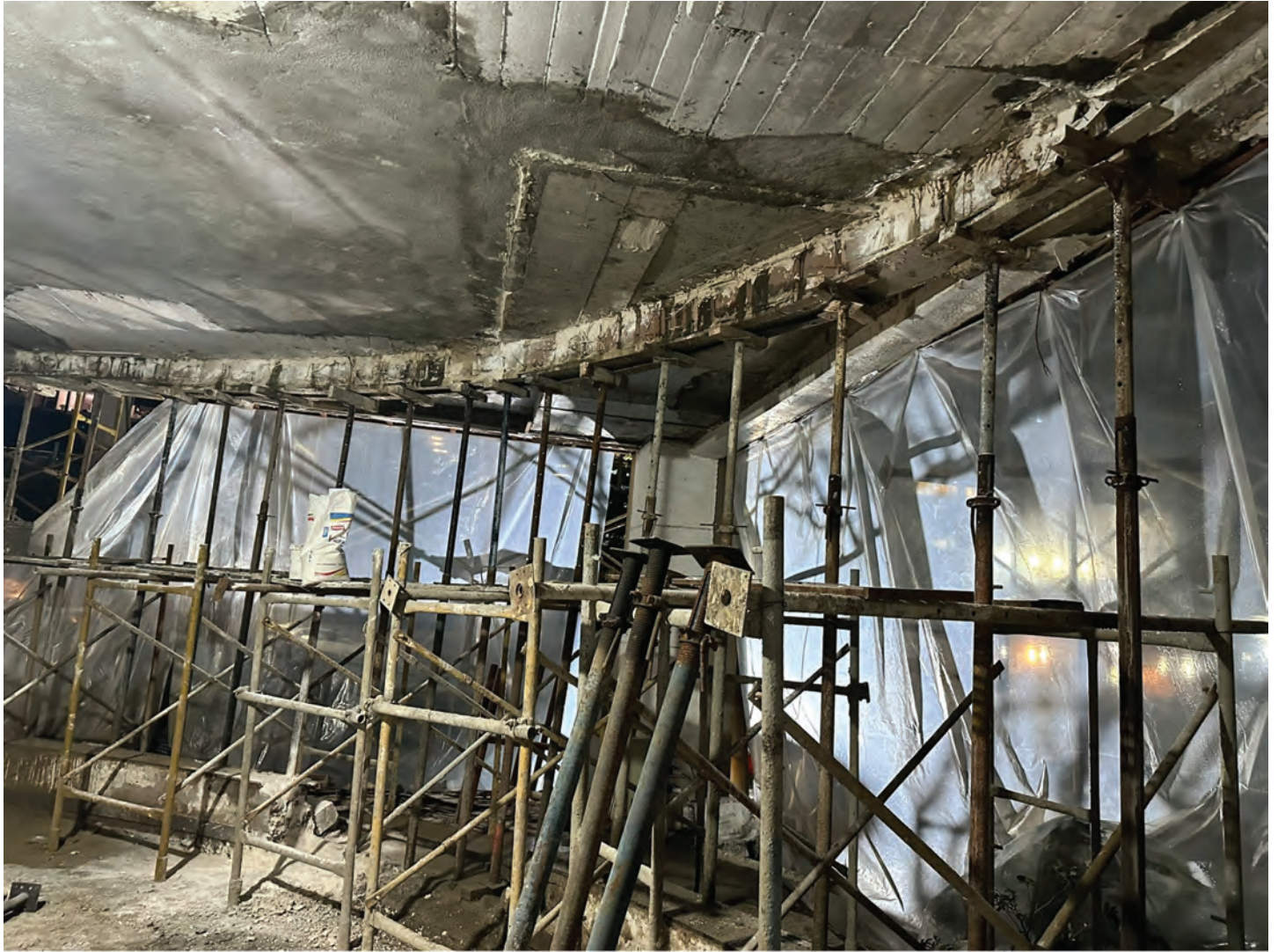
Curve Beam Made To Support The Existing Slab By Using TMT Steel Anchoring(Hilti) And Micro Concrete
