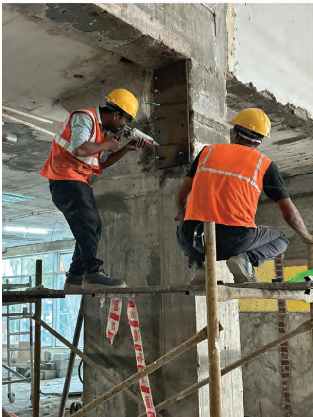
Demolished Tie Beam Strengthening By MS Beam Using Hilti Anchor Fastener & Duct Slab With Ms Fabrication Work
