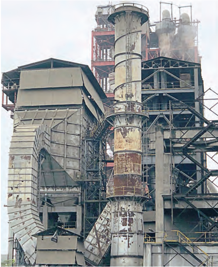
Copper Blasting And Heat Resistance Coating For MS Chimney.
