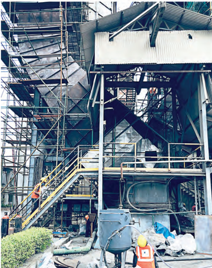
Copper Blasting And Heat Resistance Coating For MS Chimney.
