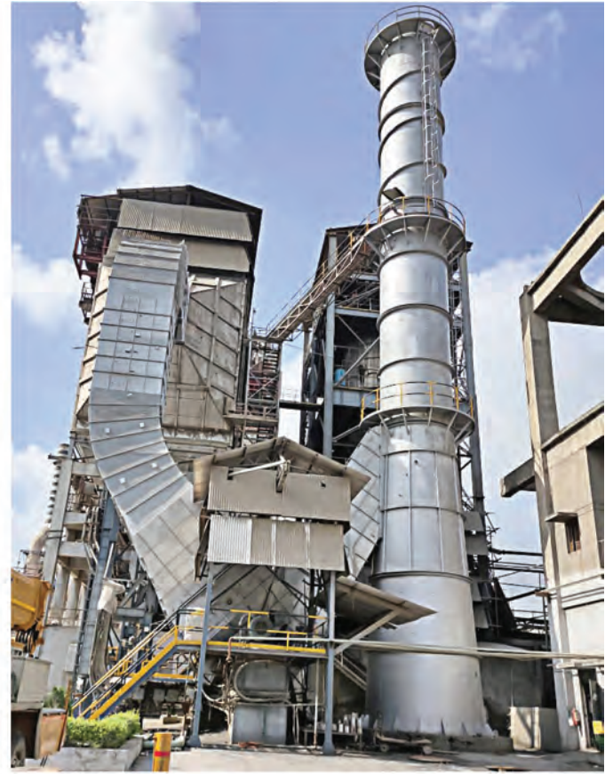
Copper Blasting And Heat Resistance Coating For MS Chimney.
