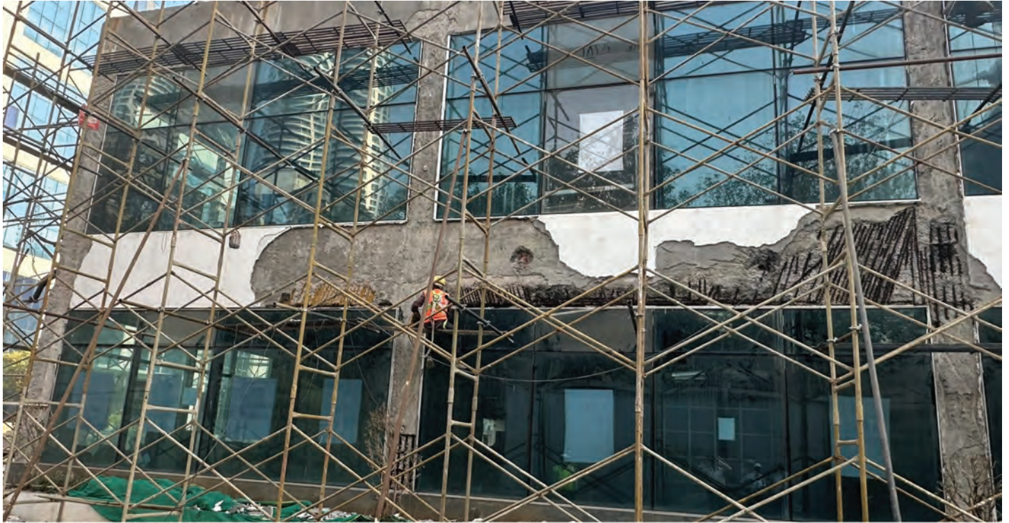
Facade Repair And Column Jacketing Work
