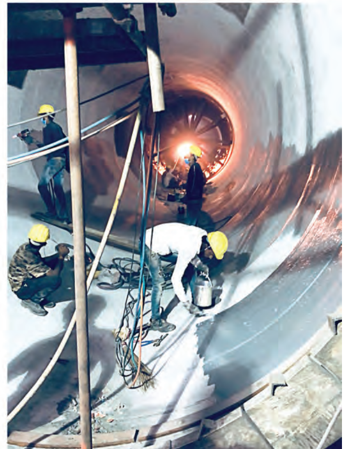
Copper Blasting And Heat Resistance Coating For MS Chimney.
