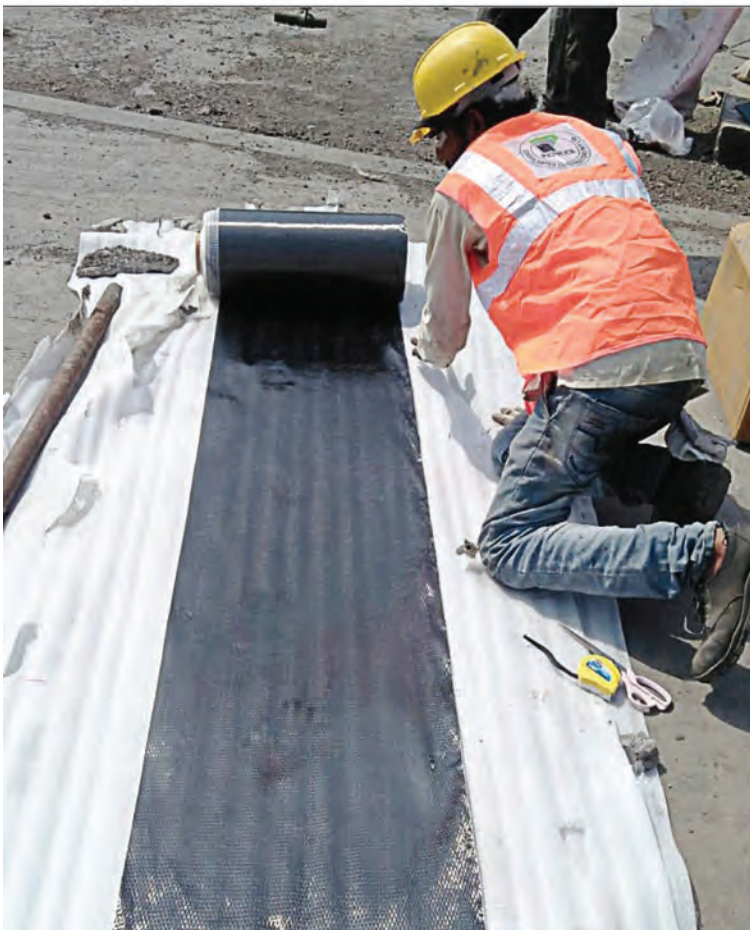
Structure Repair Work For Submerged Area Including Carbon Fiber Wrapping With Anti-carbonation Coating.
