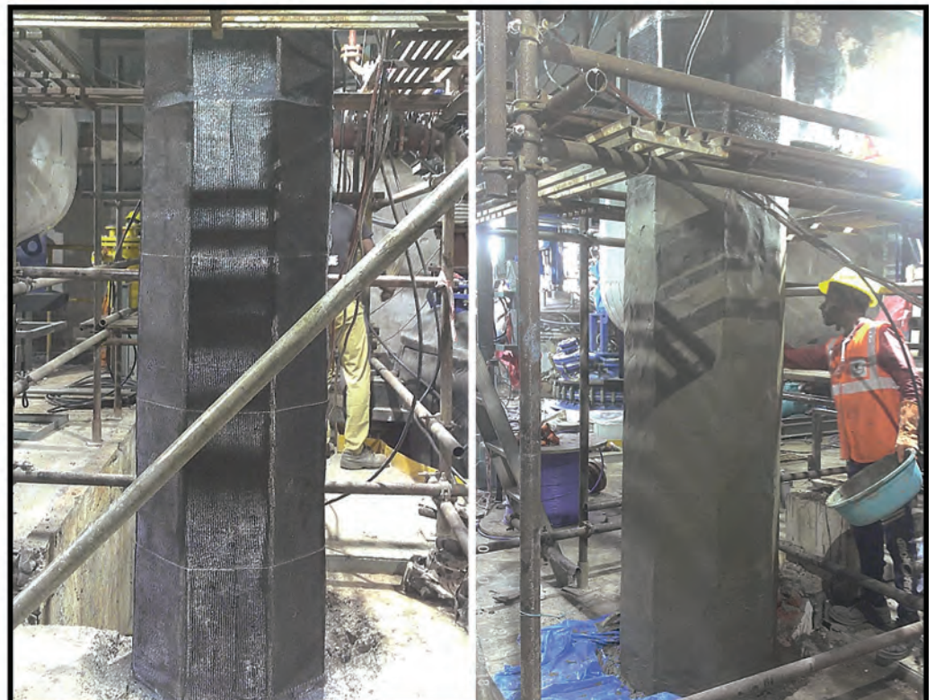
Column Strengthening Work By Carbon Fiber Wrapping With Fire Retardant Mortar
