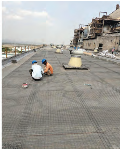
Waterproofing With Screeding Incorporating With G.I Mesh.
