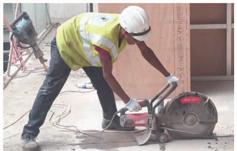
Diamond Cutting Done For Lift Shaft And HVAC Shaft
