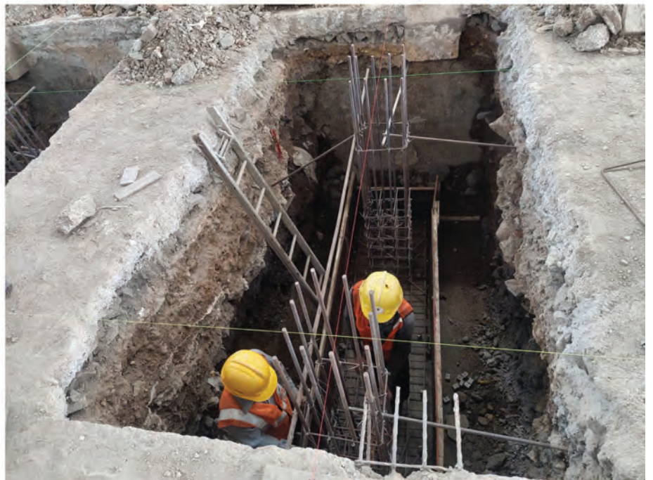
Foundation Work To Support MS Columns And Structural Member Of Ramp Connecting From Ground To First Floor.
