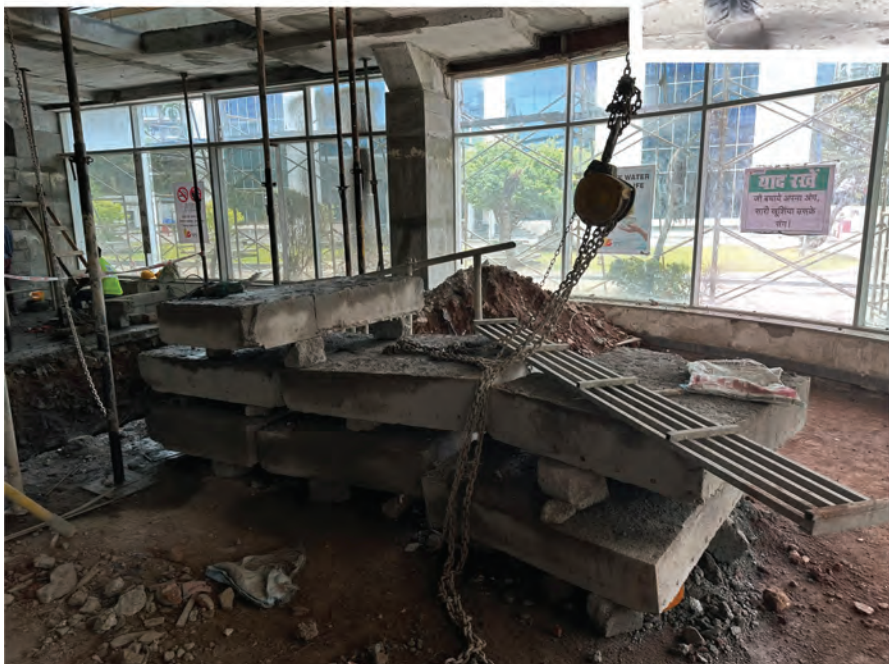
Diamond Cutting Done For Lift Shaft And HVAC Shaft
