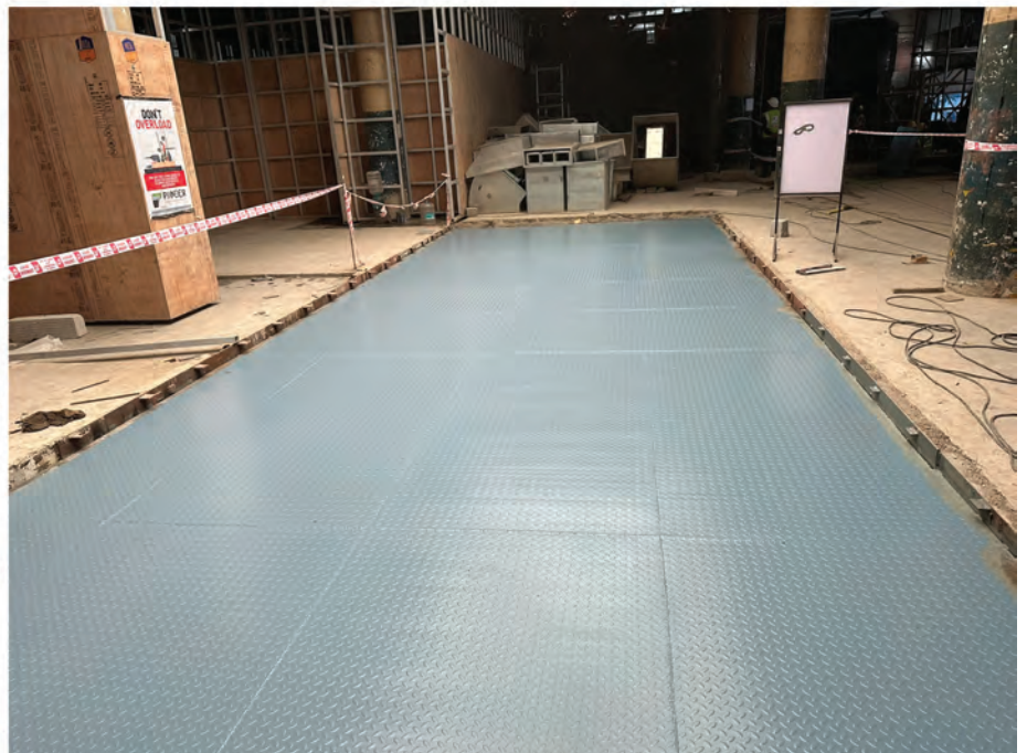
Closure Of Opening With Ms Steel Fabrication Work Finished With Anti-Corrosive Coating.
