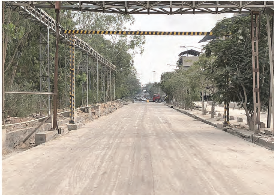
Trimix Road In Industrial Area With Floor Hardener Coating.
