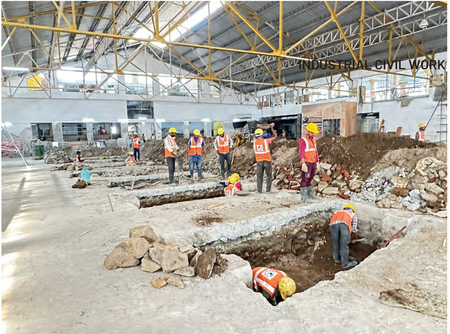
Foundation Work To Support MS Columns And Structural Member Of Ramp Connecting From Ground To First Floor.
