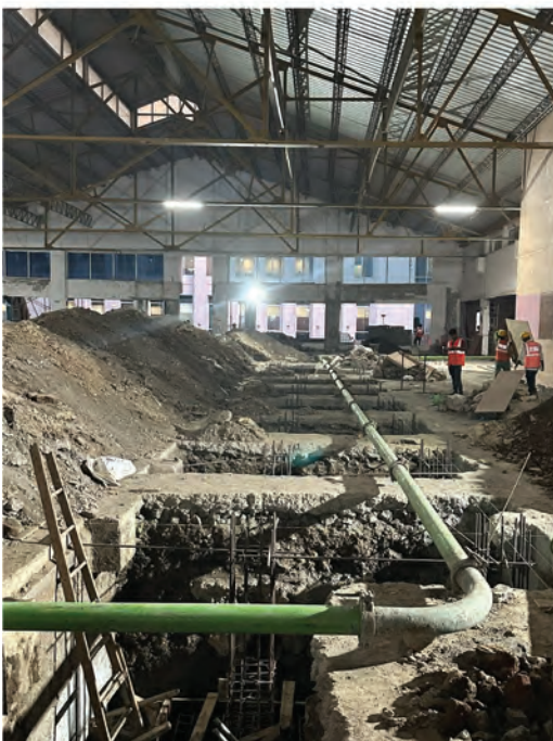
Foundation Work To Support MS Columns And Structural Member Of Ramp Connecting From Ground To First Floor.
