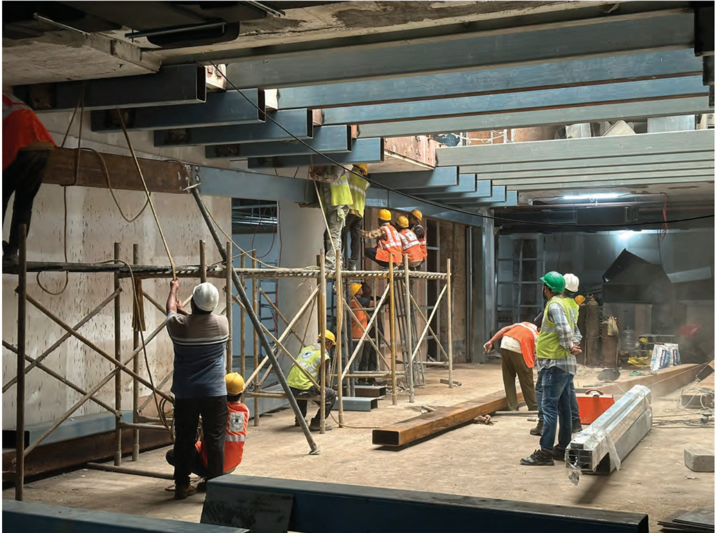
Closure Of Opening With Ms Steel Fabrication Work Finished With Anti-Corrosive Coating.
