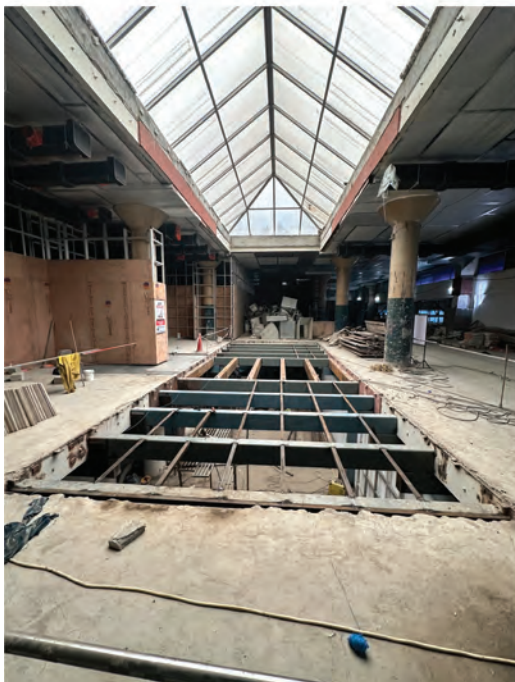
Closure Of Opening With Ms Steel Fabrication Work Finished With Anti-Corrosive Coating.
